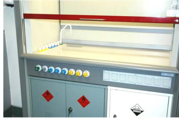
Fume Cupboard service outlets
