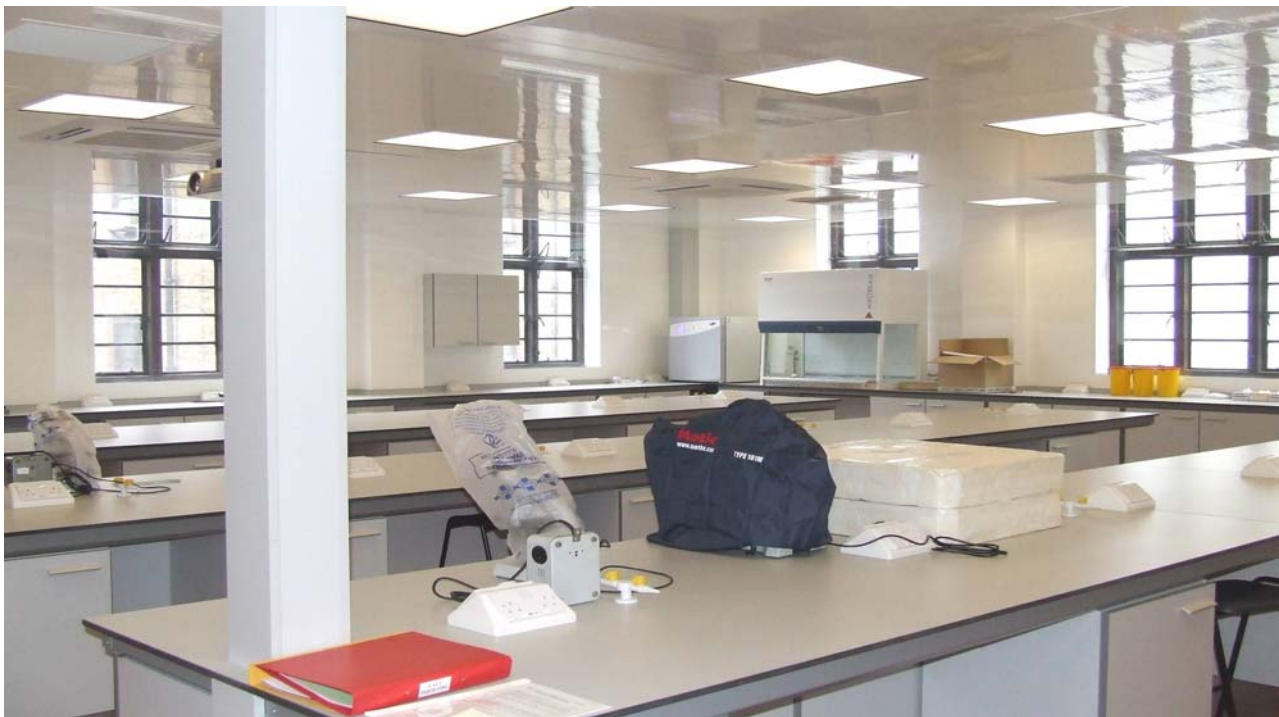
Island and perimeter benching
